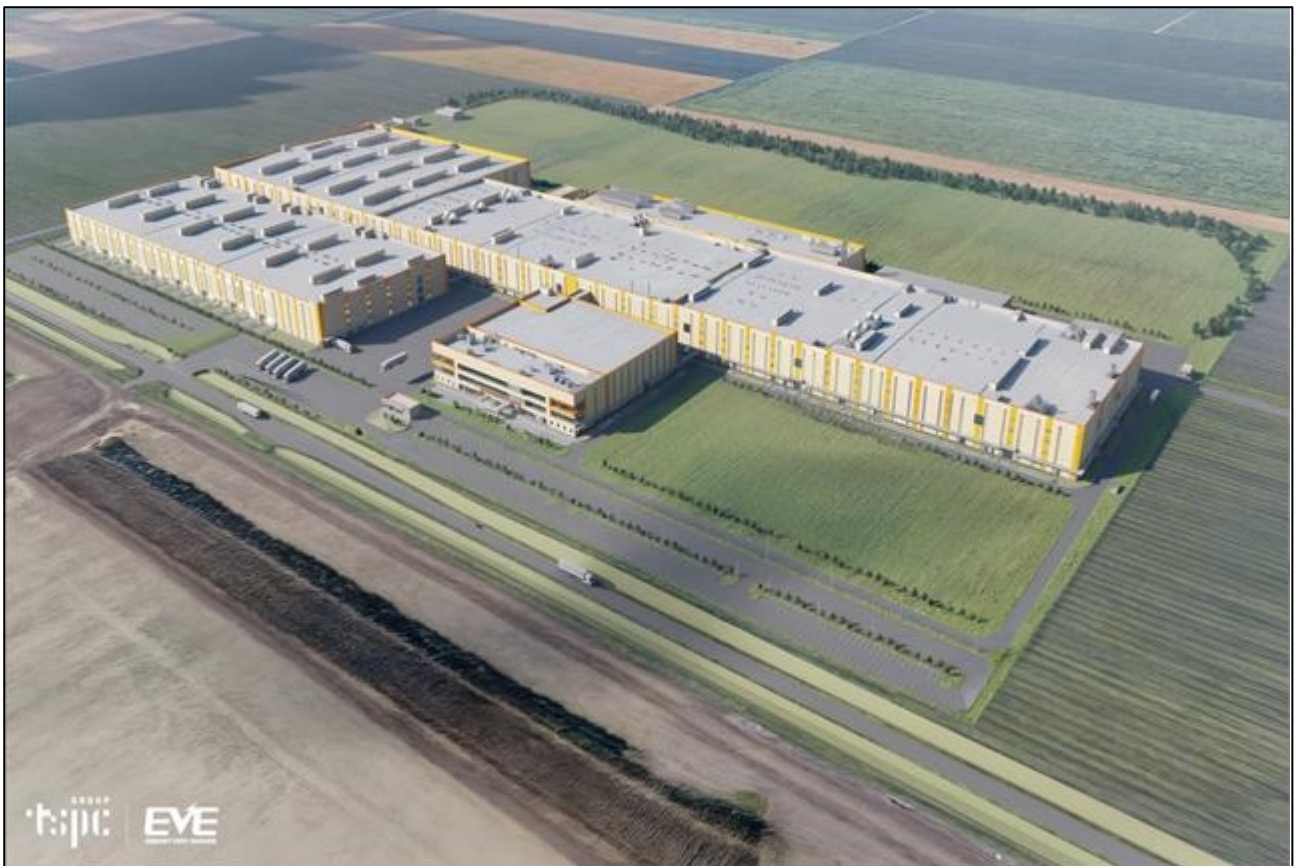
30. Figure 3: Three-dimensional appearance of the factory buildings and the structure of the building and its landscape manifestation as seen from the southeast.
